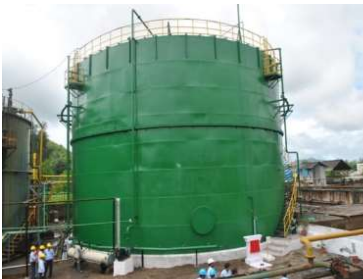
Biogas Scrubbing and Cleaning System
